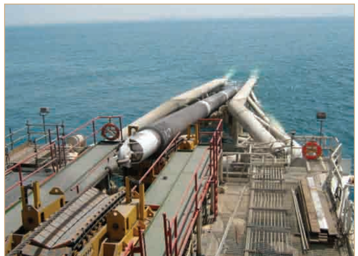
Laydown of the 34 inch pipeline in progress
